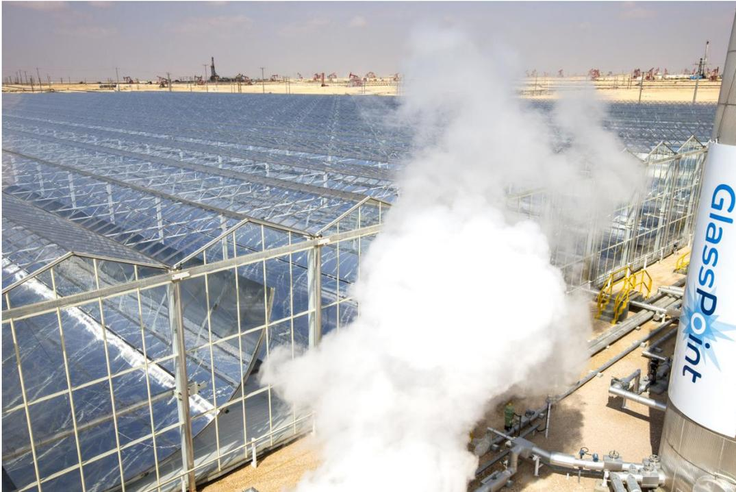
Figure 5. Glasspoint solar steam generators at the Amal West oilfield [29].
